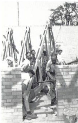
WORKERS PREPARE TO LIFT A ROOF TRUSS INTO POSITION
