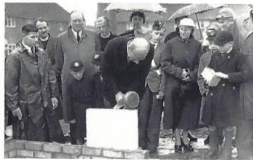
REV. D. H. HICKS, AREA SUPERINTENDENT, LAYING A FOUNDATION STONE, JUNE 1956
