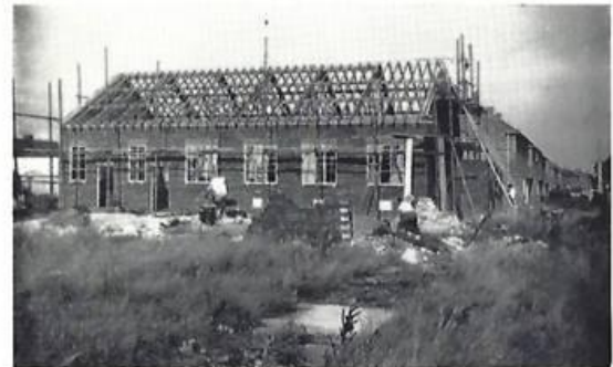
COMPLETING THE FRONT GABLE, SEPTEMBER 1957
